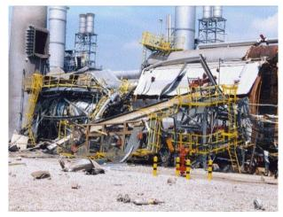
At 0220 hours, technicians reportedly used the diesel burner, which resulted in Master Fuel Trip and Shut-Off the fuel systems completely. Hence, LPG burner was chosen to restart which was unsuccessful during the initial attempts. A bypass procedure was used by the commissioning team in their attempt to restart the boiler which resulted in explosion.
